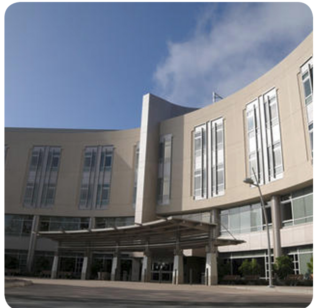
El Camino Women's Hospital - Mountain View, CA
